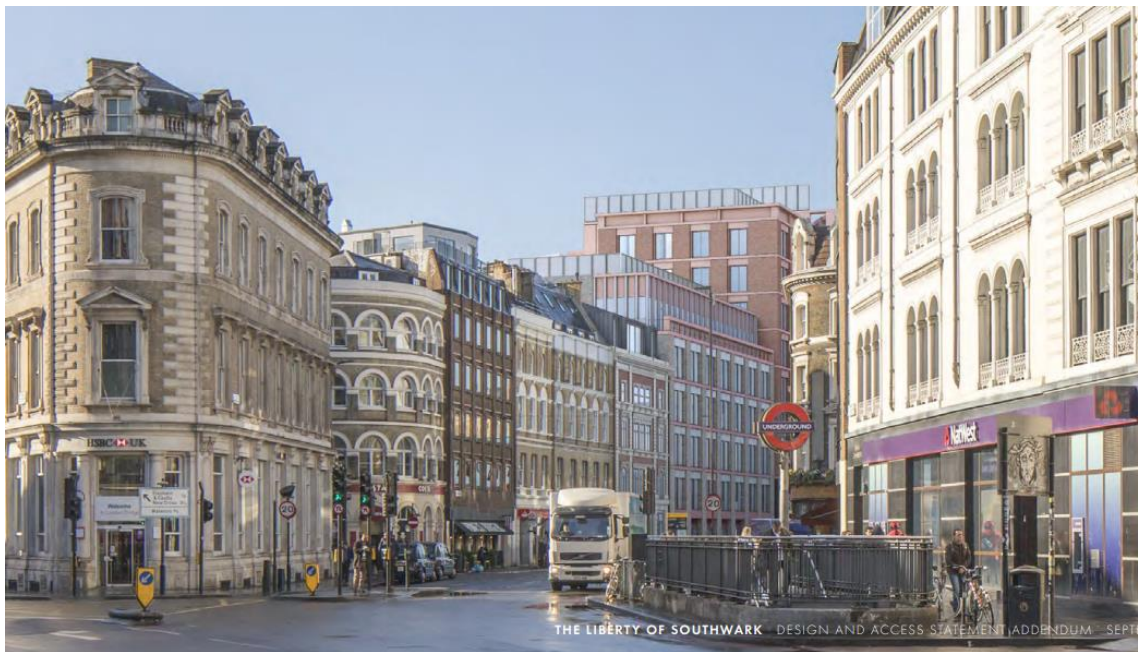
View west along Southwark Street
